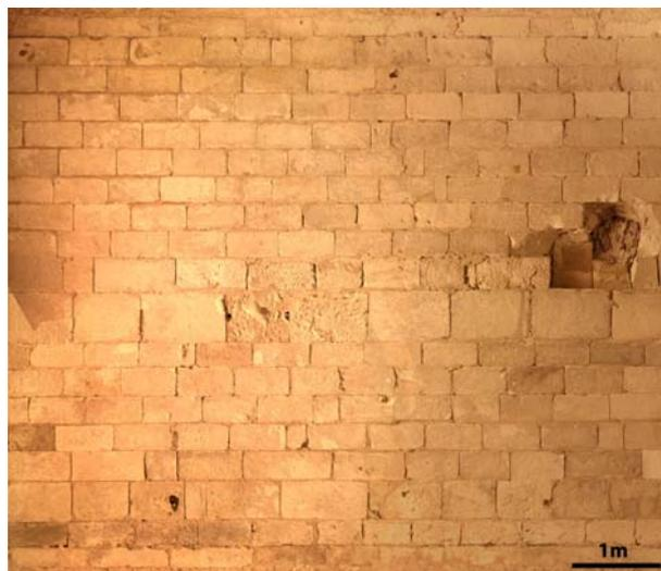
Figure 5: Unwrapped orthoimage of the second room vault.
